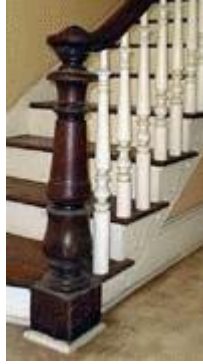
Newel post and balusters, first floor staircase
