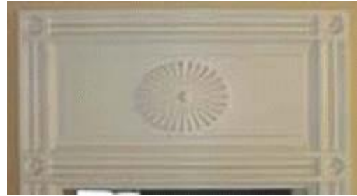
Detail, first floor doorway
