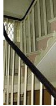
Balusters, third floor staircase
