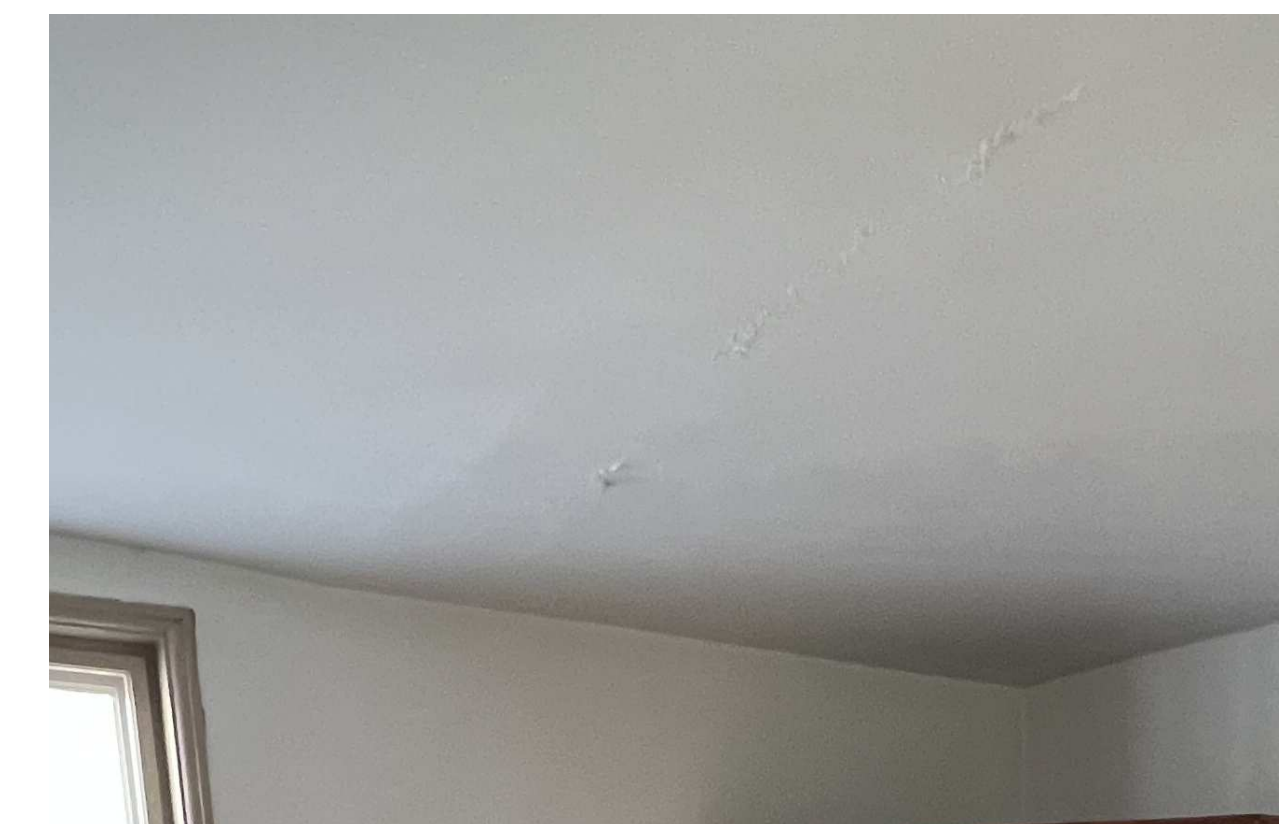
EAST CEILING PLASTER
