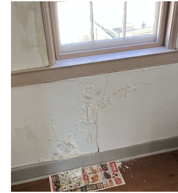
NE WINDOW PLASTER
